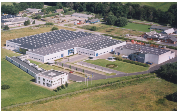
A NorthWest Air Photo of the new factory
