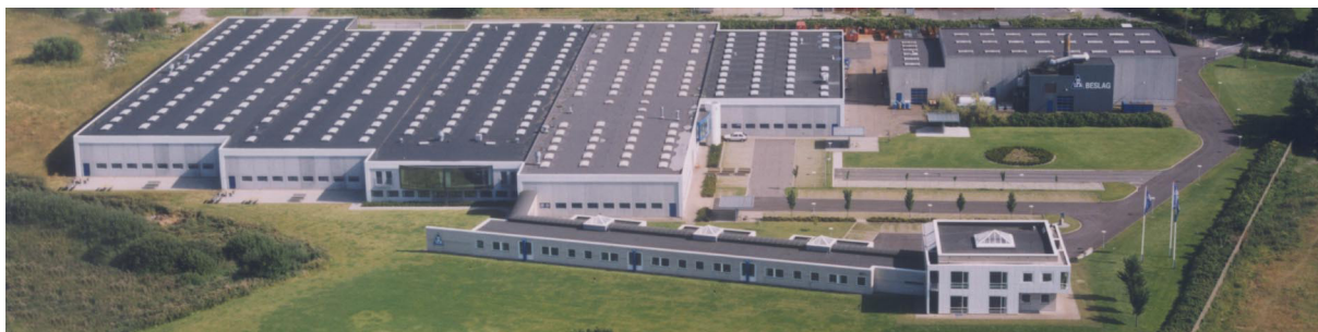
IPA - New factory with the new production facilities
